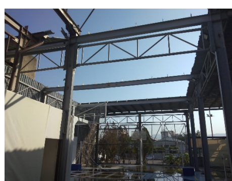
Available Space for additional solar panels
