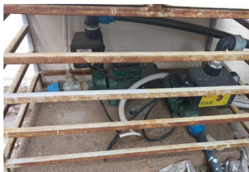
1.5hp booster pump (operational) & 0.5hp booster pump (redundant)
