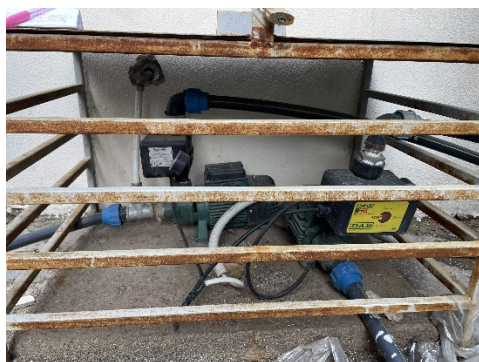
1.5hp booster pump (operational) & 0.5hp booster pump (redundant)
